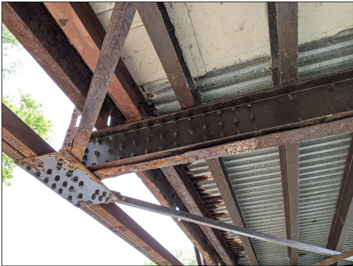
Typical Repaired Floor Beam
