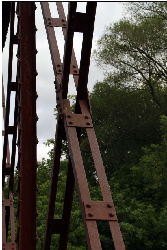
Figure 25 diagonal bracing
