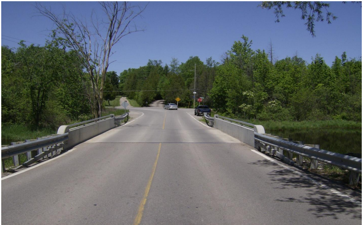
Railing Option 2 – Concrete Parapet Wall with Steel Railing
