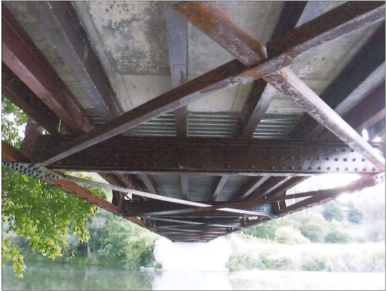
Figure 28 underside of bridge showing extensive repairs - K. Smart Associates photo
