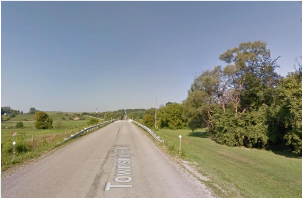
Figure 2b: View, looking east, atop a bridge located along Township Road 11, near Ayr, ON. This bridge appears to be constructed in a similar manner to that planned for the Bridge Street Bridge. This structure appears to include a gradual incline of the road upwards towards the bridge, likely completed to accommodate the seasonal flooding typical within the Nith River.
