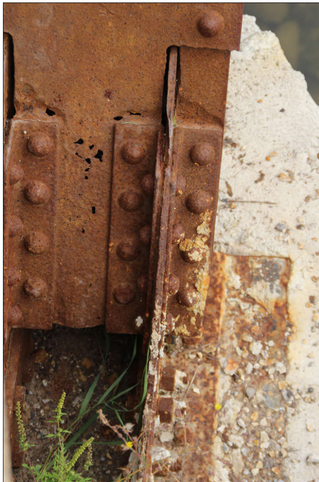
Figure 22 deteriorated end post to abutment connection
