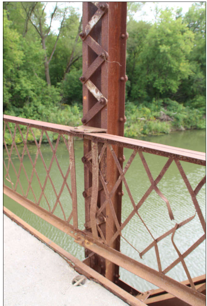
Figure 23 V-laced vertical member &amp; damaged railing
