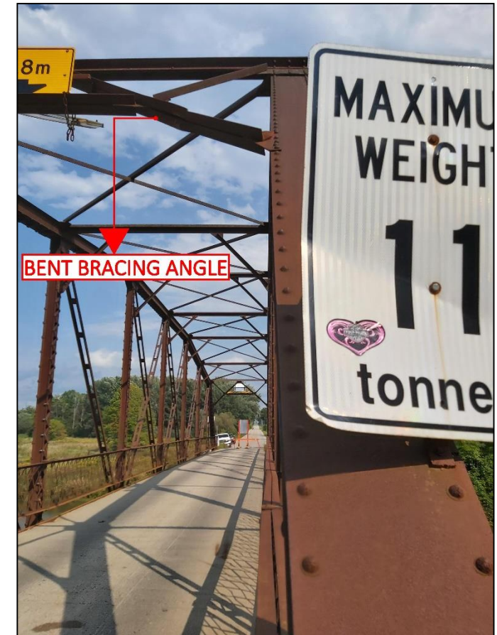
The latest road closure started from mid-September 2021 due to vehicular collision with the overhead bracings. Note one of the bent bracing angles in picture above.
