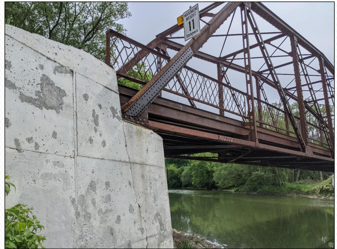
Typical Repaired Truss Chord
