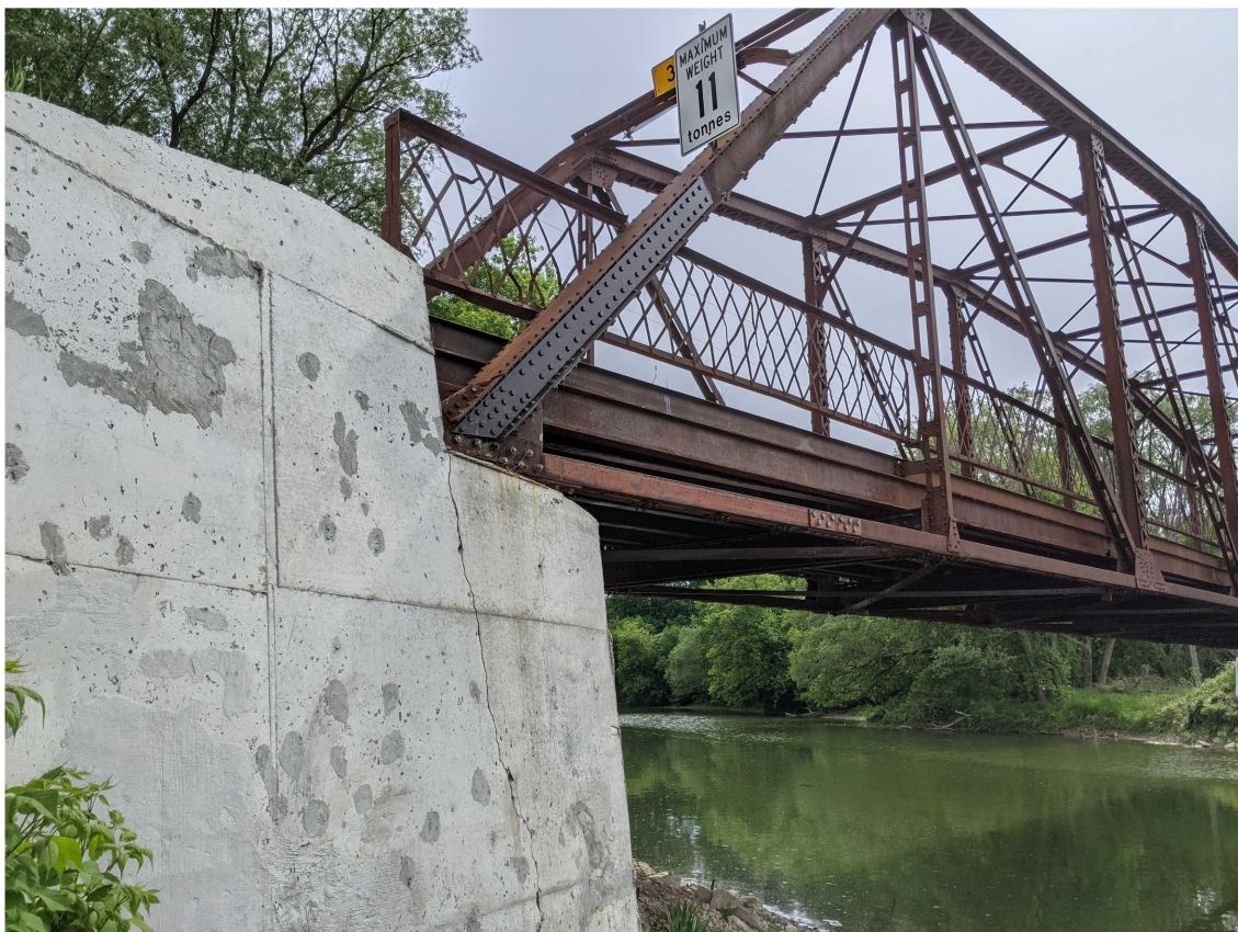
10. Typical Repaired Truss Chord
