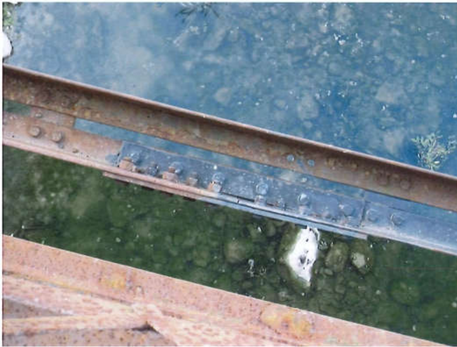
Photo 7: Repairs at bottom chord
