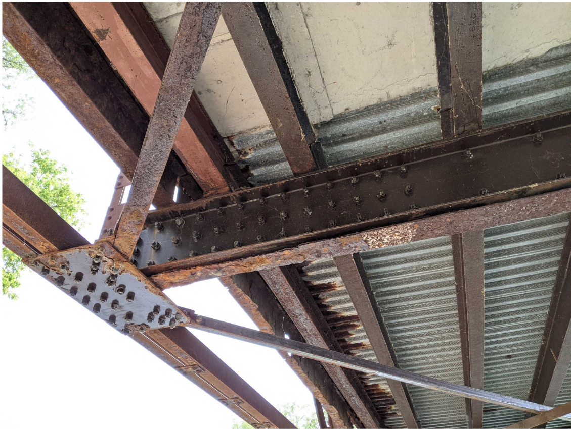
9. Typical Repaired Floor Beam
