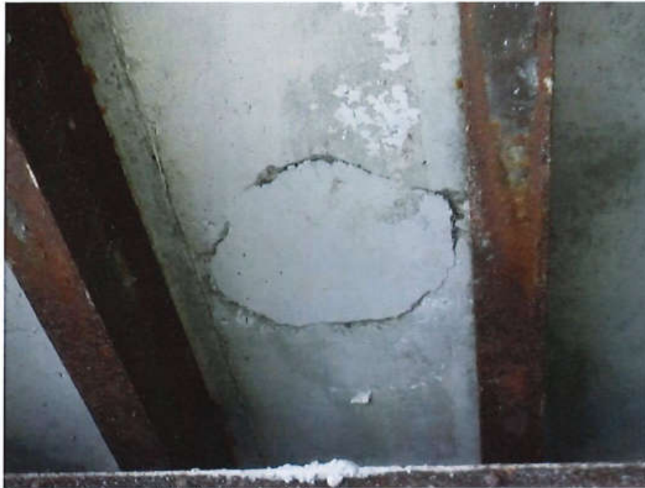
Photo 9: Severe delamination at soffit interior
