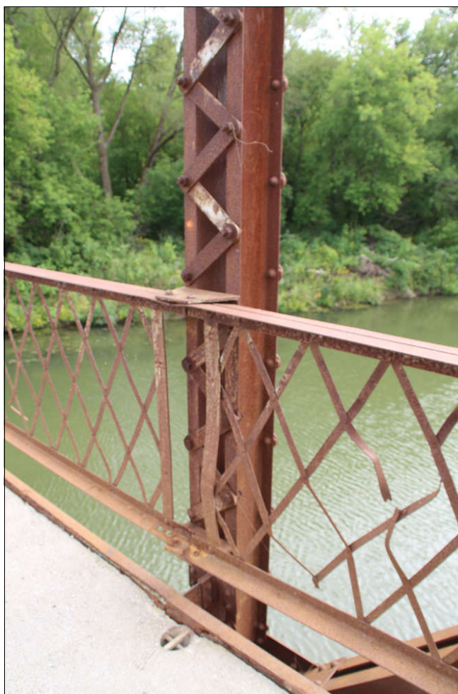
Figure 23 V-laced vertical member &amp; damaged railing
