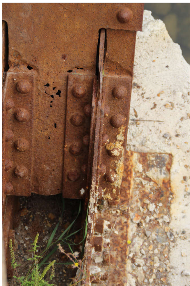
Figure 22 deteriorated end post to abutment connection
