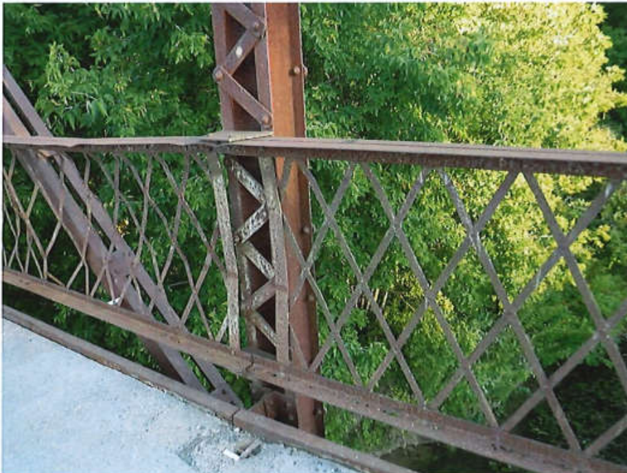
Photo 6: Substandard railing system over structure
