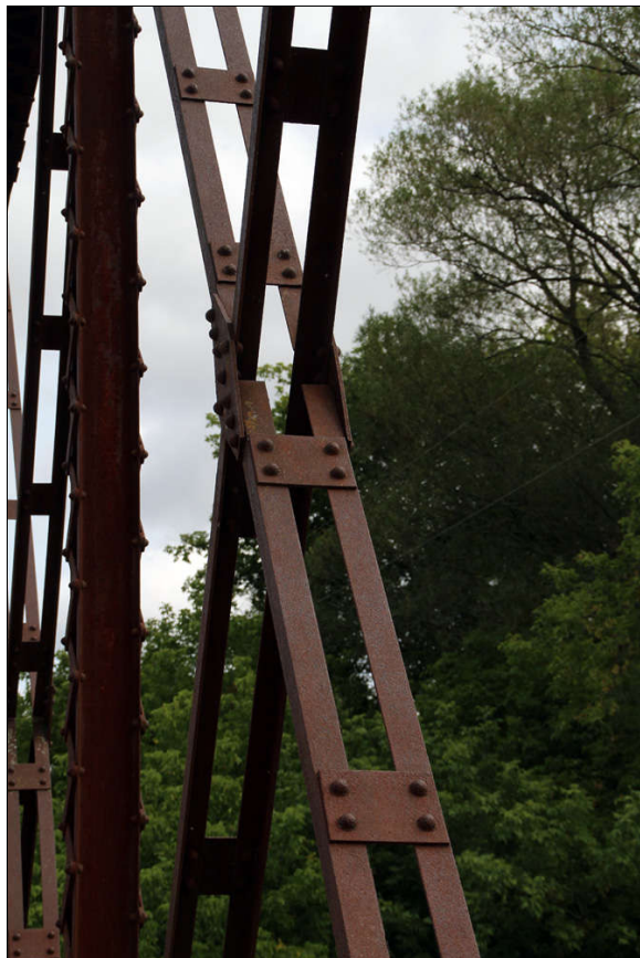
Figure 25 diagonal bracing
