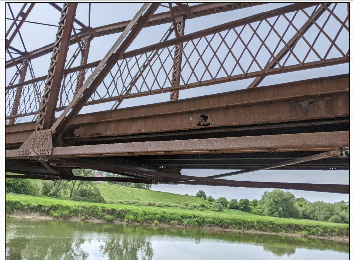
Typical Perforated Stringer
