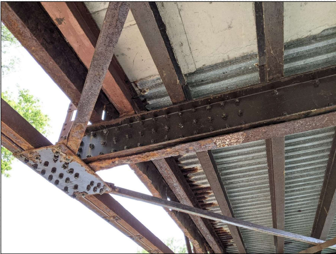
Typical Repaired Floor Beam
