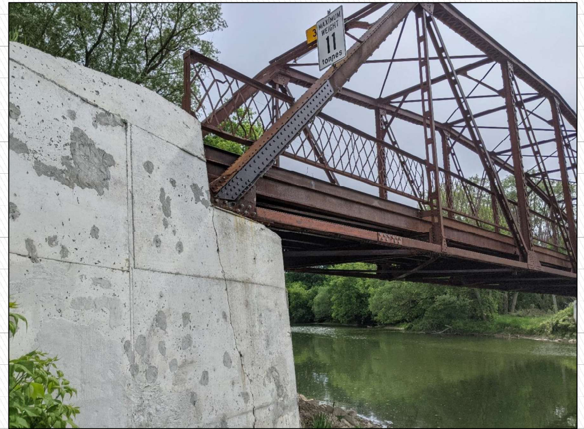
Typical Repaired Truss Chord
