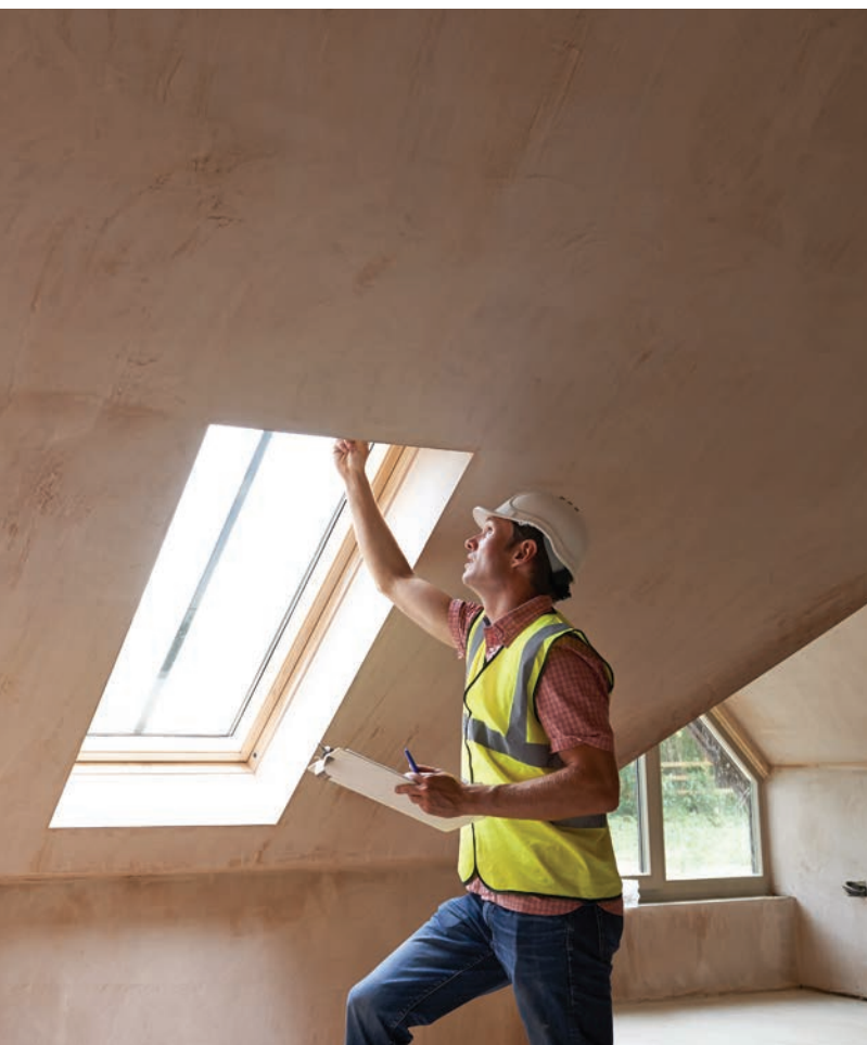
Figure 9: A municipal building inspector
