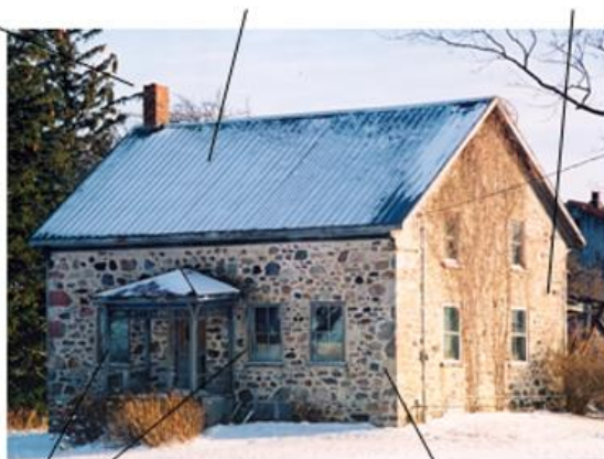
Irregular Placement of Windows
