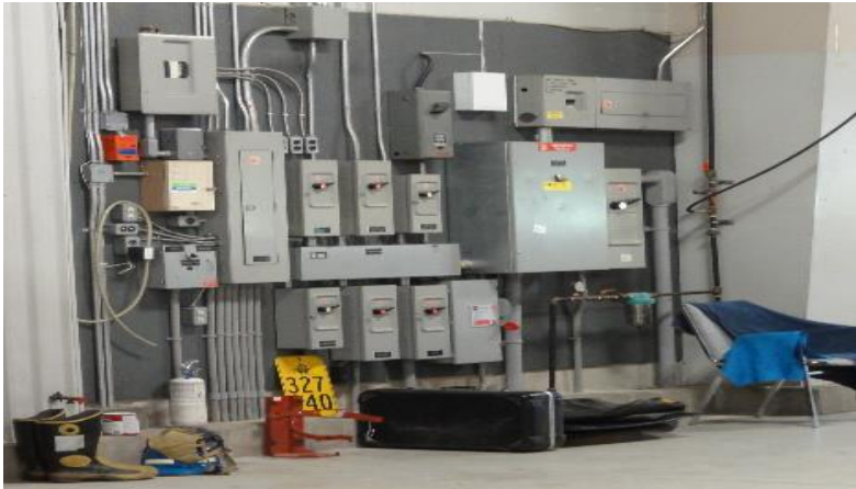
Photograph: water protection for electrical panel required.
