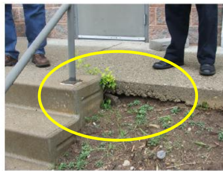
Photograph: Sidewalk erosion on west elevation.
