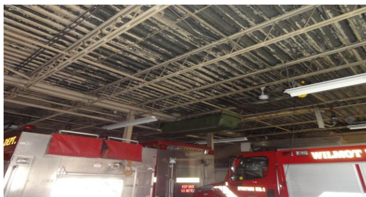
Photograph: peeling paint over apparatus floor.
