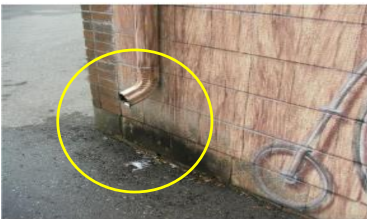
Photograph: Voids in the foundation and no splash pad for downspout noted.
