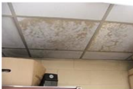
Photograph: Staining of ceiling tiles.
