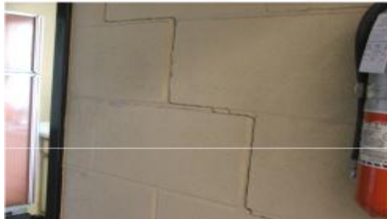
Photograph: Cracked masonry in interior wall
