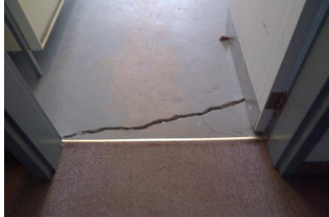
Photograph: Crack in concrete floor by training room
