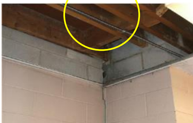
Photograph: Wood joist conditions and masonry wall separation at the chimney.
