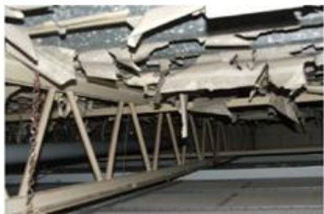
Photograph: Peeling paint on roof framing.
