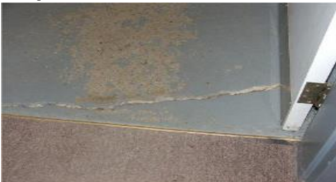
Photograph: Subsidence issues noted through a portion of the structure.
