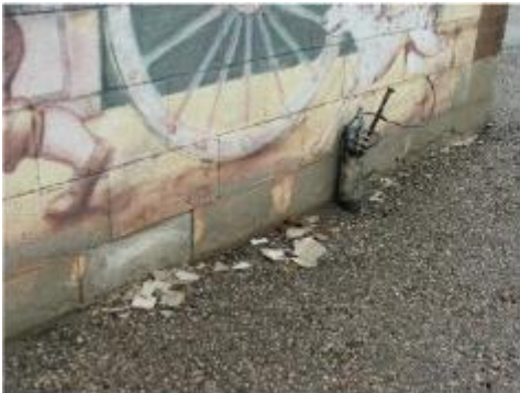
Photograph: Parging on exterior damaged.
