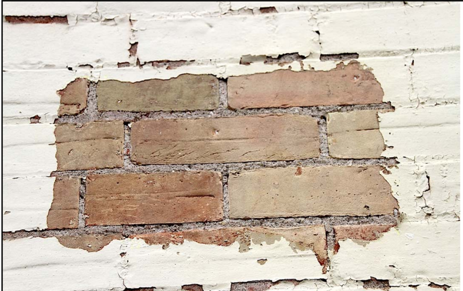
After a third application, the original bricks appear. Note the grout
