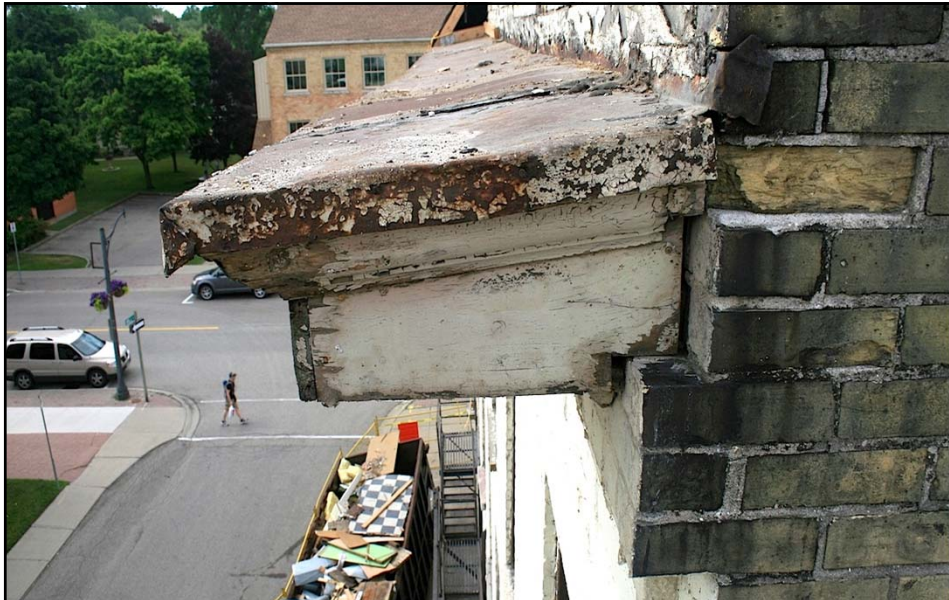
The parapet uncovered with original tin cap
