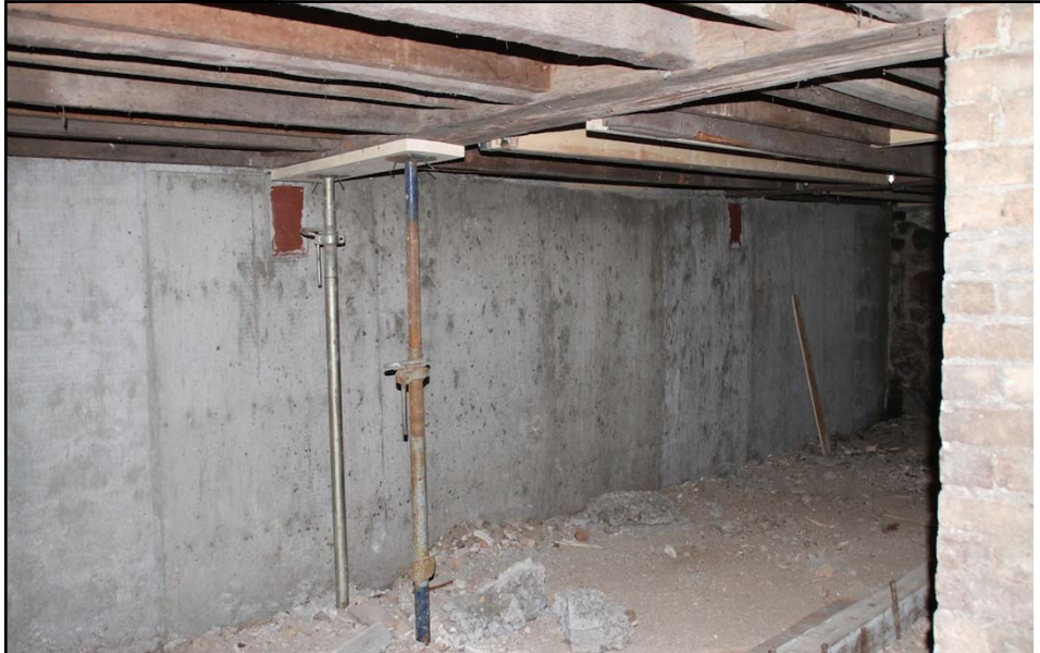
New walls have been poured around perimeter of the original basement
