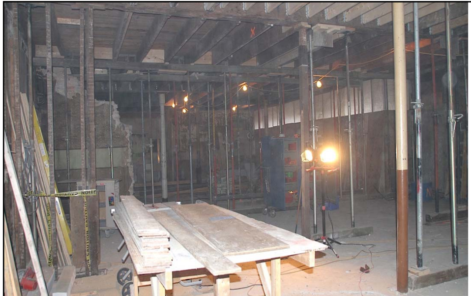
Main floor with all the temporary steel posts
