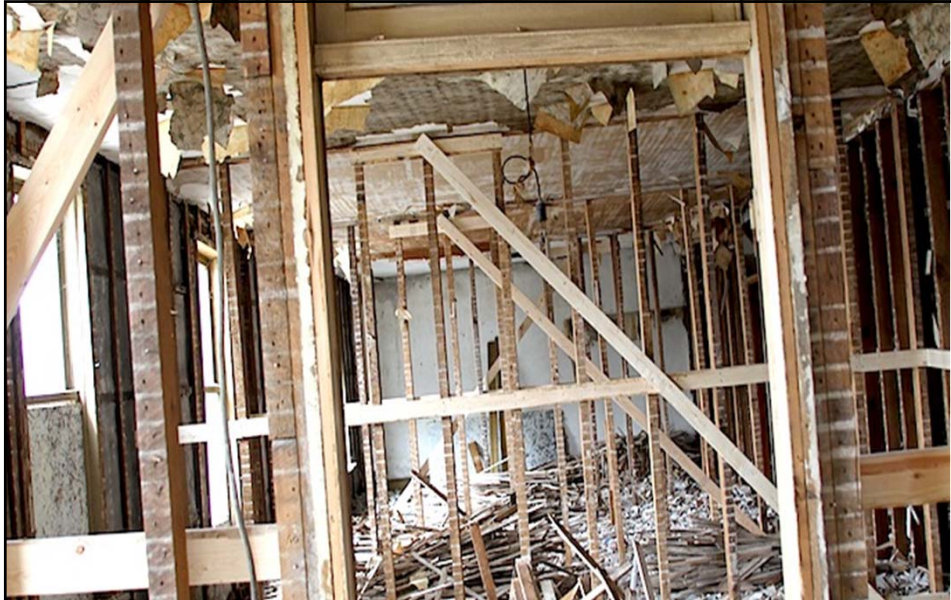
Lath and Plaster removed
