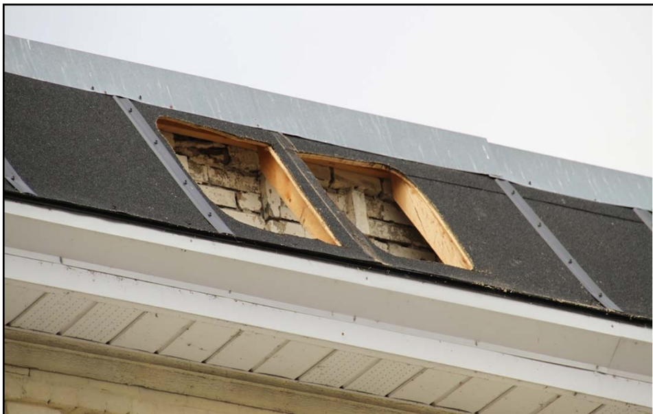
#4 Uncover the Parapet
