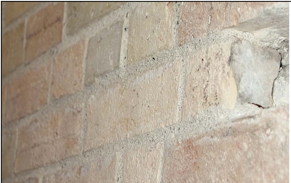
#6 All the grout had to be removed and reapplied on the original building
