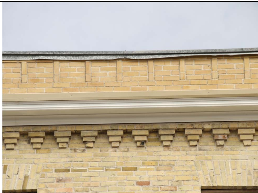
Replaced parapet bricks and cornice
