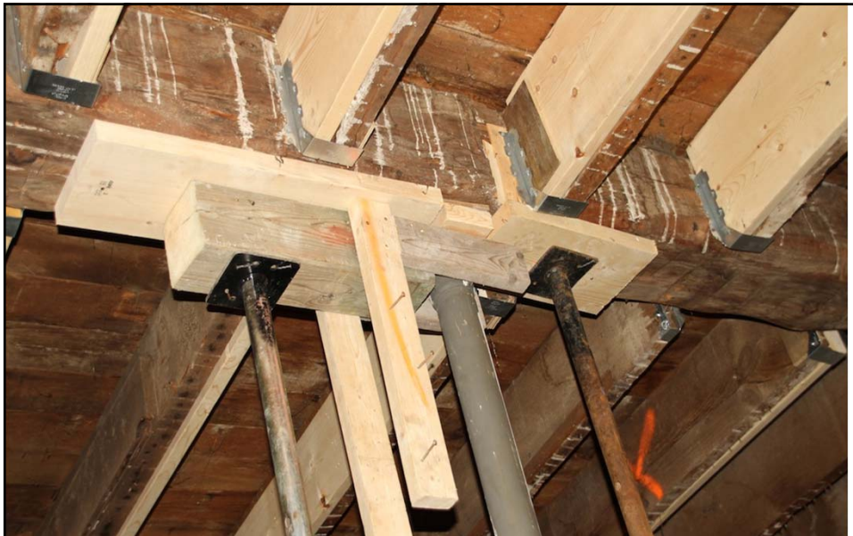
Braced under key areas on the main floor for the 6" sag of the floor
