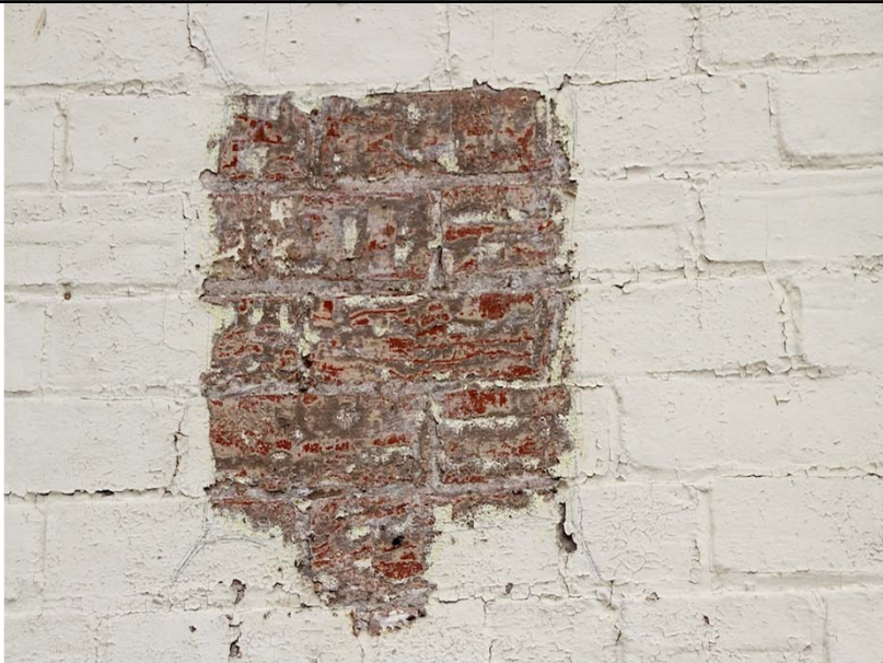
#5 Clean Bricks: To remove 3 coats of cream paint, we used Peel-Away. After one application, most of the yellow paint was removed.
