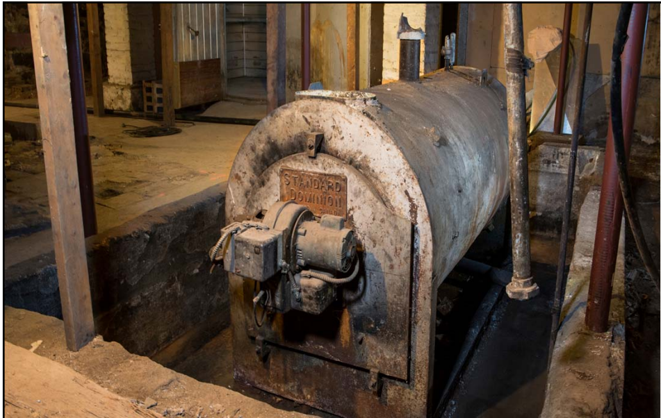
A post was removed for boiler installation in 1908 and never replaced
