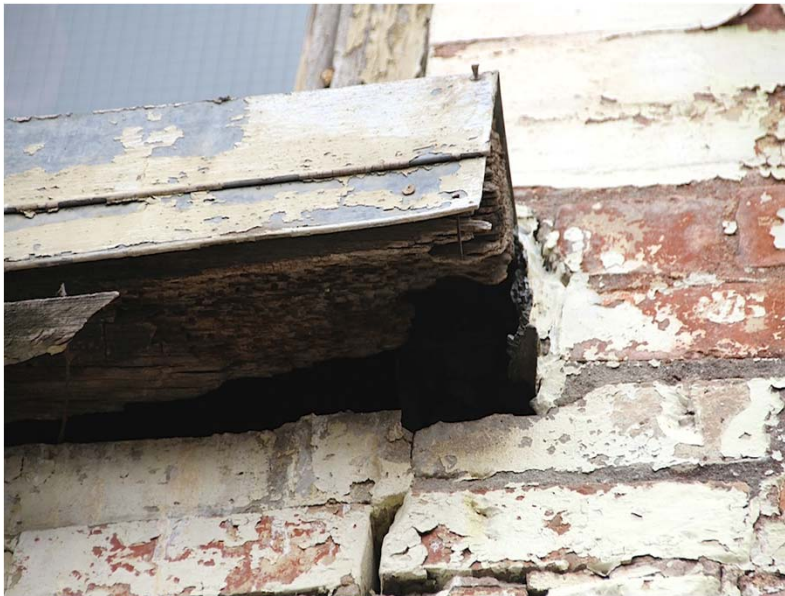
#2 All window sills have to be replaced due to old age and rot
