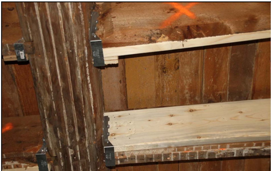
Reinforced joists that had been mortised into the beams
