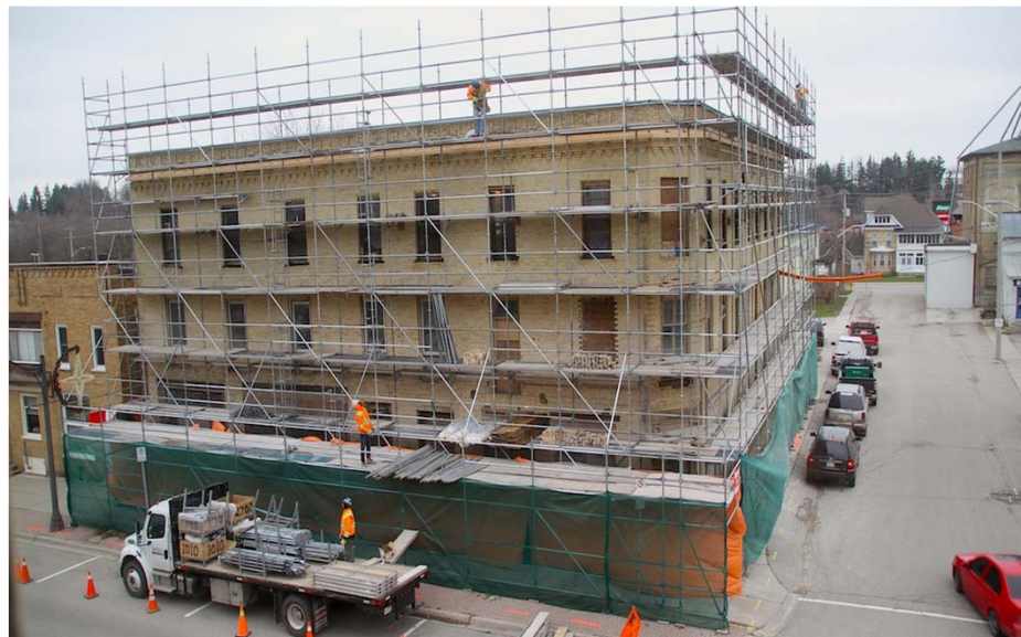
#7 We replaced over 7,500 bricks + parapet
