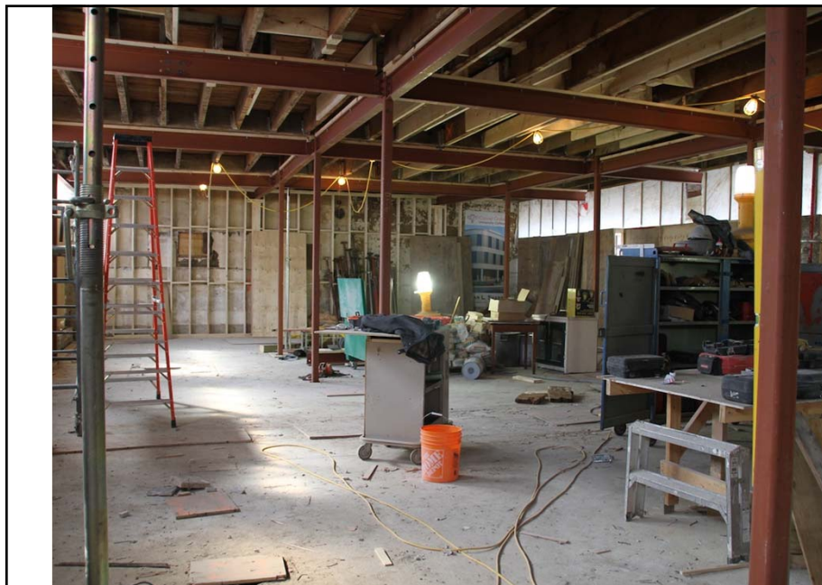
Main Floor with 29 steel beams and 13 steel posts
