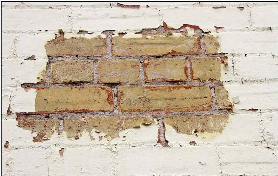
After a second application, most of the red stain was removed
