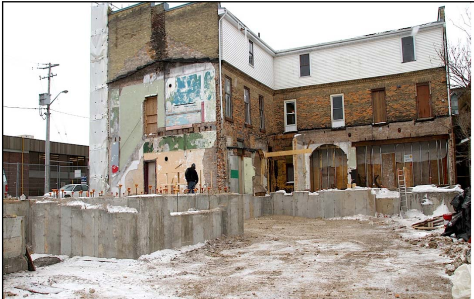
March 30, 2015 Foundations for the addition and kitchen are complete
