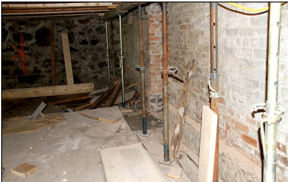
Added temporary structural posts in basement
