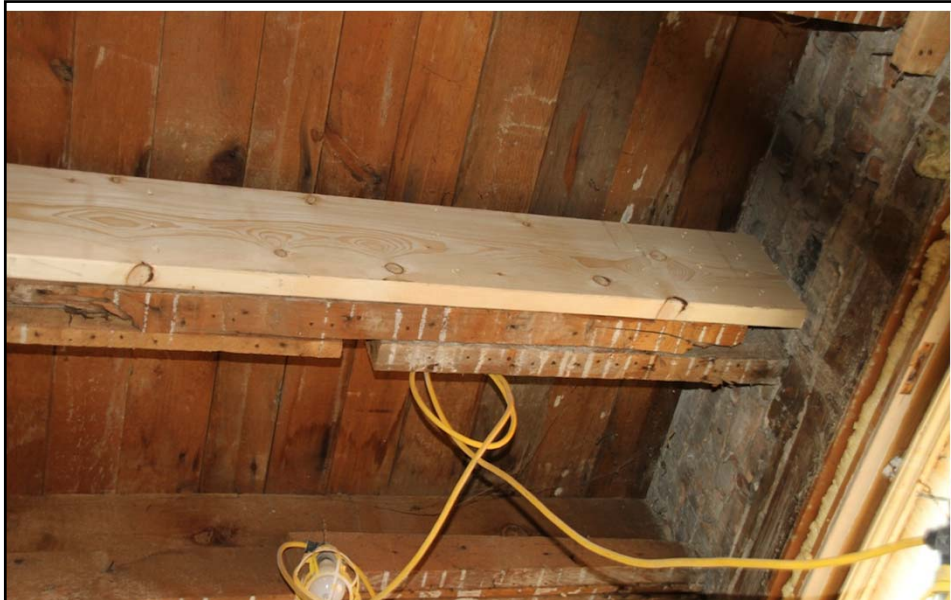
#8 A tiny problem emerged with overall lack of structural support - sistering
