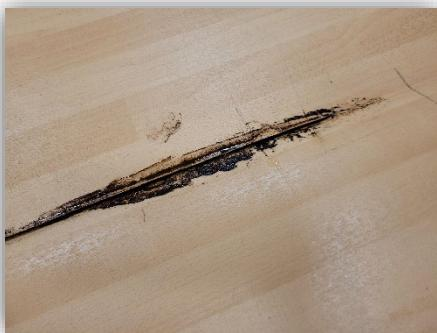
The significant challenges posed by the current flooring condition necessitate complete replacement rather than a restoration approach. The entire flooring system must be removed and disposed of offsite. The old underlayment must also be completely eliminated, involving the use of solvents and potentially grinding the surface to expose the concrete subfloor. This process is essential to create a porous surface that allows for proper adhesion of the new flooring adhesive.
